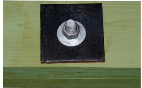
Typical HBPS58 Installation
